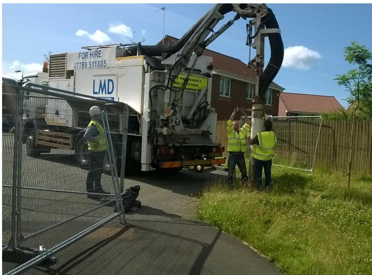
What better solution than to hire an industrial vacuum truck (see picture below) to clear the pipe?
